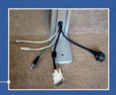
For larger sized cables, a cable trough (cable support) can be installed. A feedthrough base is used for carrying cables to the floor.
